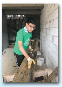
Carlos carefully bends a steel bar using a machine Carlos小心使用工具,把鋼條折彎
